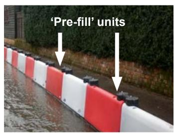
Insert connection keys ensuring each key is fully inserted. The base of each connection key should be in full contact with the ground. Correct insertion can be valiadated in one two ways:
